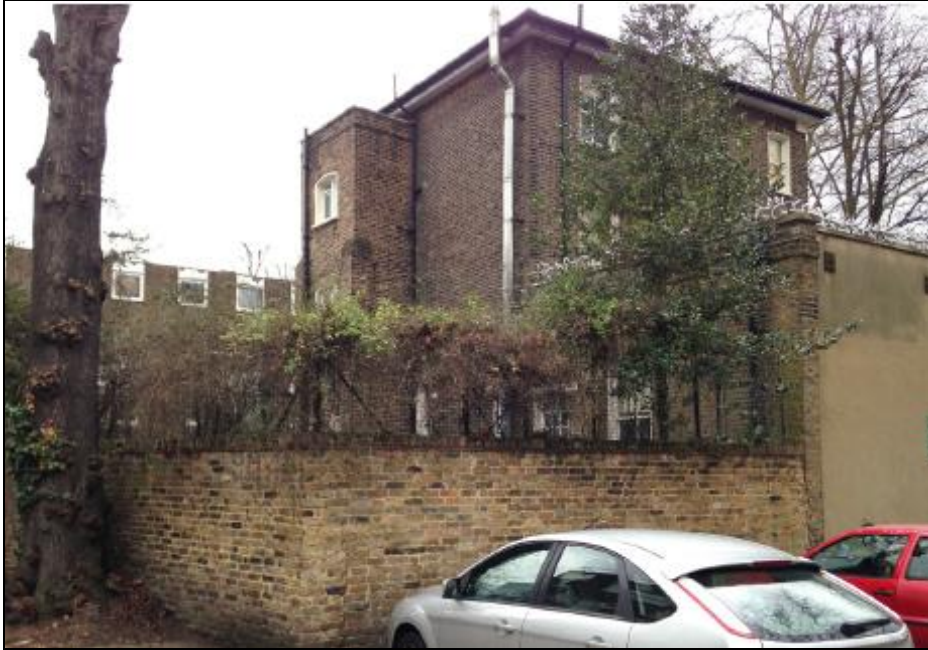
Image 2: Rear elevation from adjoining residential parking
